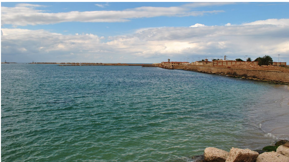
The low lying coastlines of Africa, like Alexandria here, are vulnerable from rising sea levels caused by climate change. Image by the EES.
