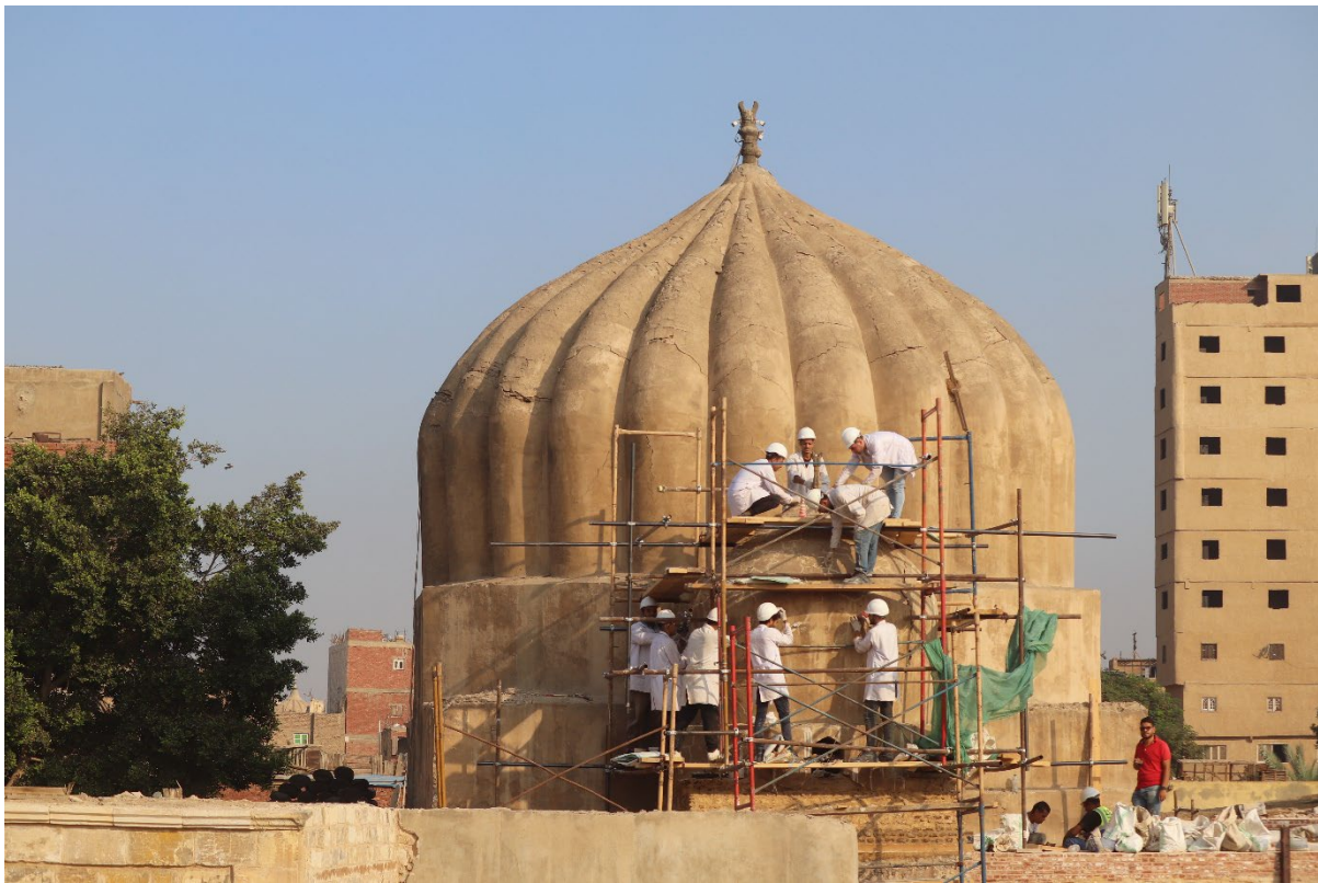
Conservation works on the main dome of Yahya al-Shabih. Image Megawra-BEC.
